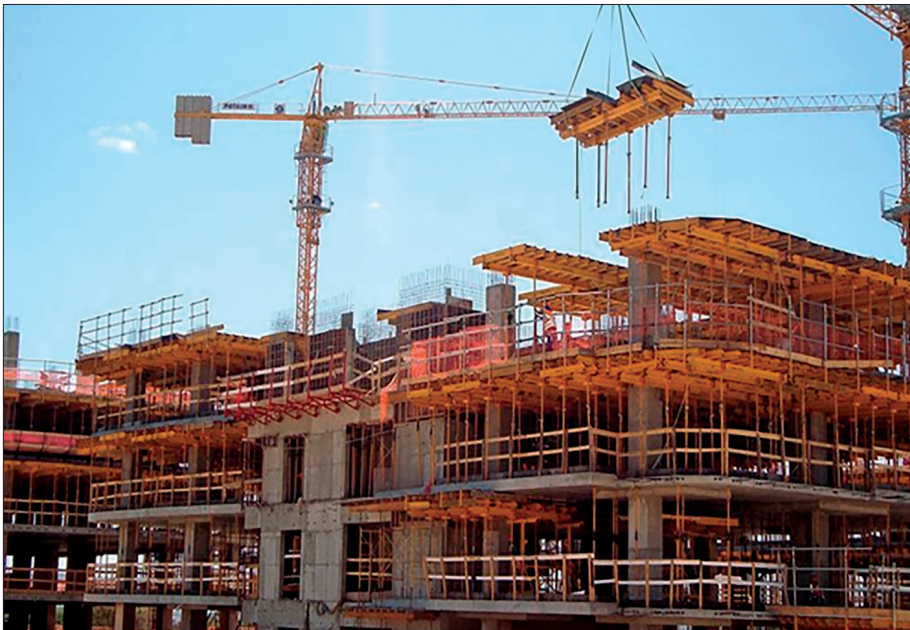
Figure 2. Flying forms system: (b) overall view.
