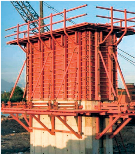
Figure 4. Jump forms system: (b) overall view of a septum's formwork.
