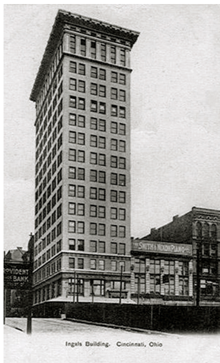
Figure 1. Ingalls Building (Cincinnati, Ohio, 1903).
