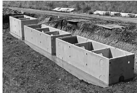
Figure 3. Settling tanks.
